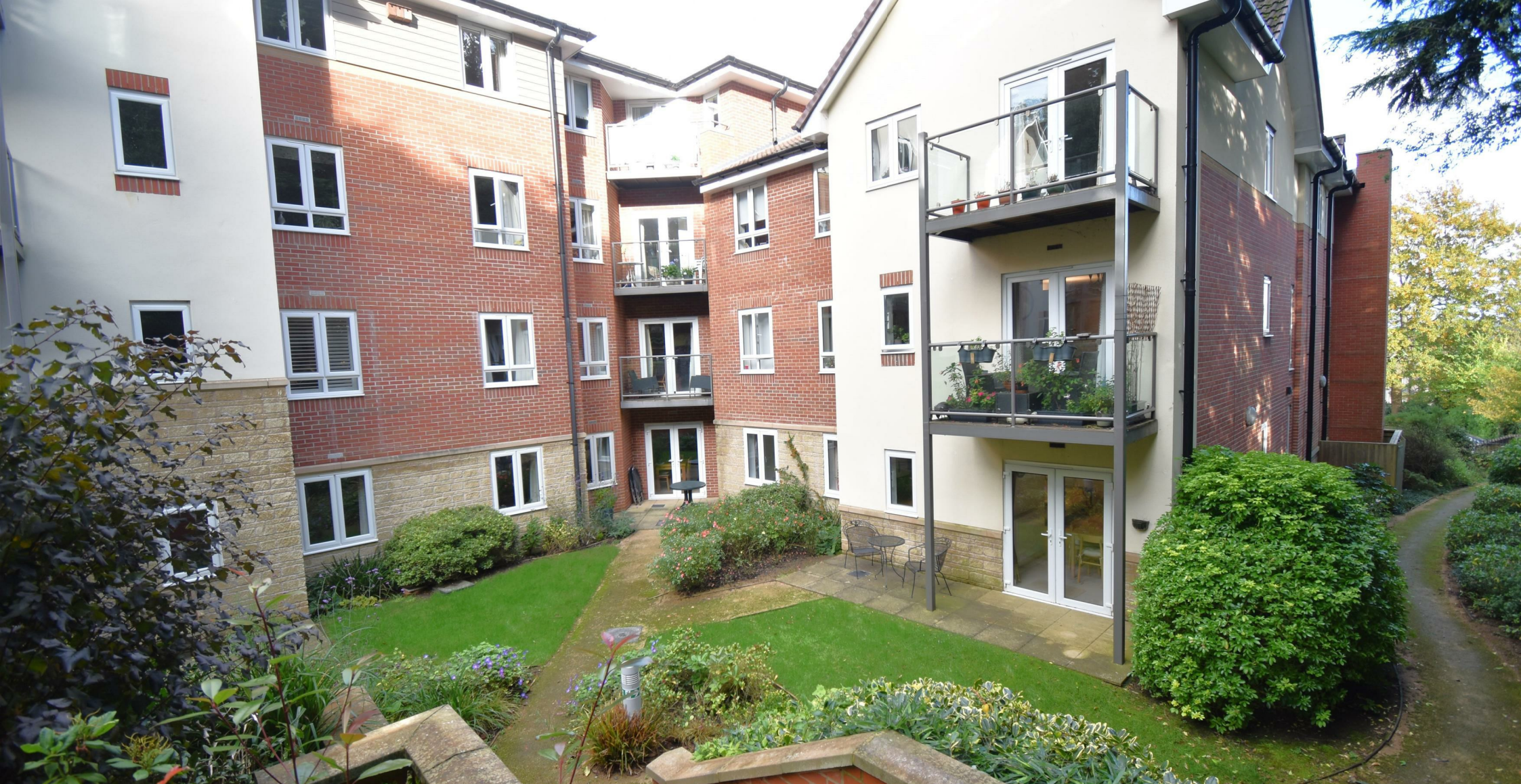
APARTMENT 3, ADLINGTON HOUSE, SLADE ROAD, PORTISHEAD, BS20 6BB
